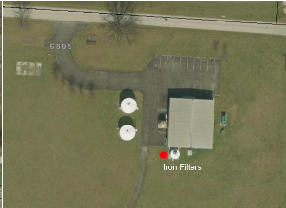
Little Walnut Water Treatment Plant
