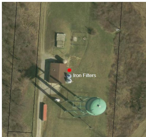
Greenfield Water Treatment Plant
