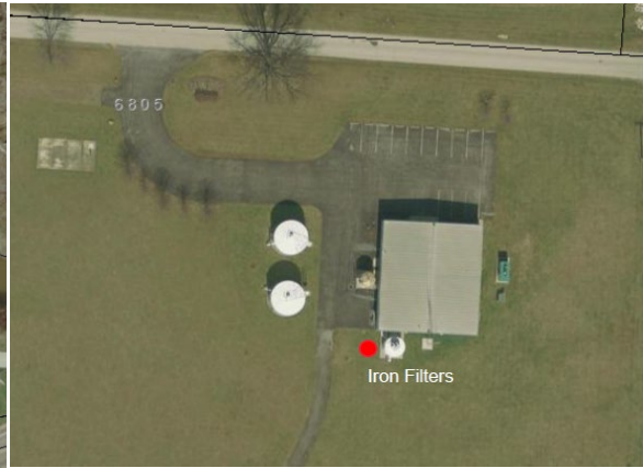
Little Walnut Water Treatment Plant
