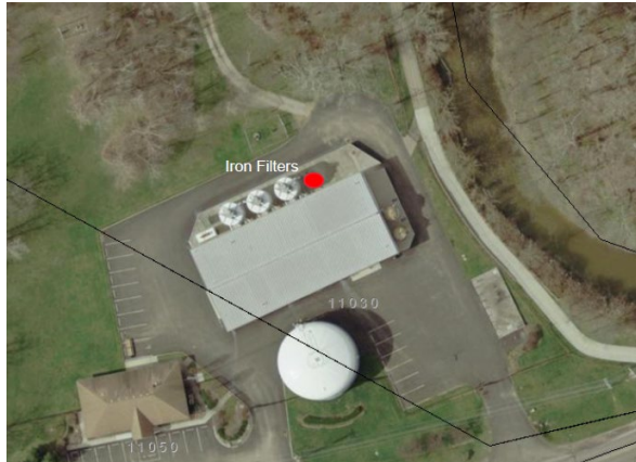
Tussing Road Water Treatment Plant
