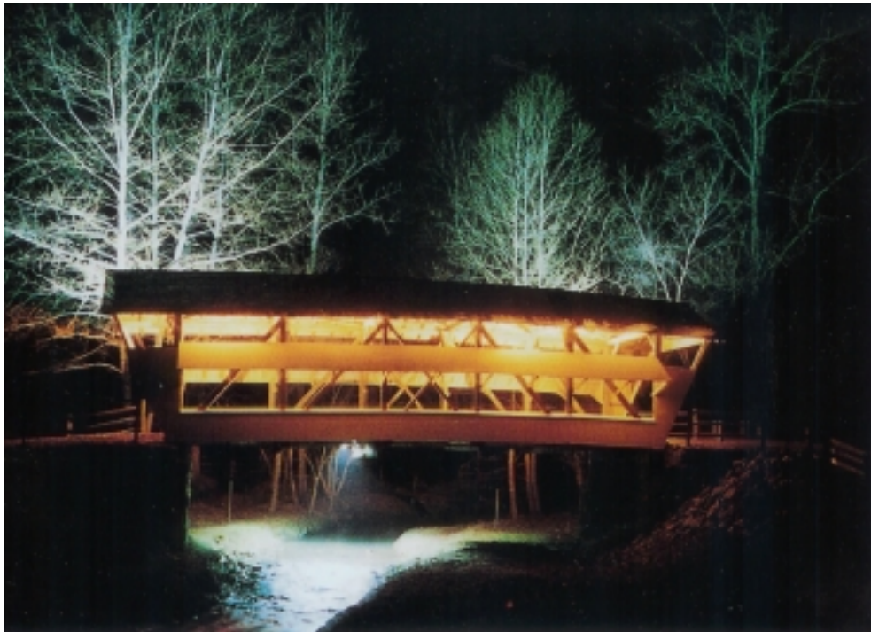
Mink Hollow Covered Bridge
