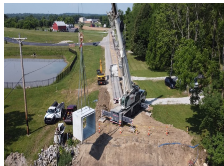
County forces replaced a culvert on Carroll-Eastern Road with a reinforced concrete box, widened shoulders, and replaced guardrail (pictured above).
