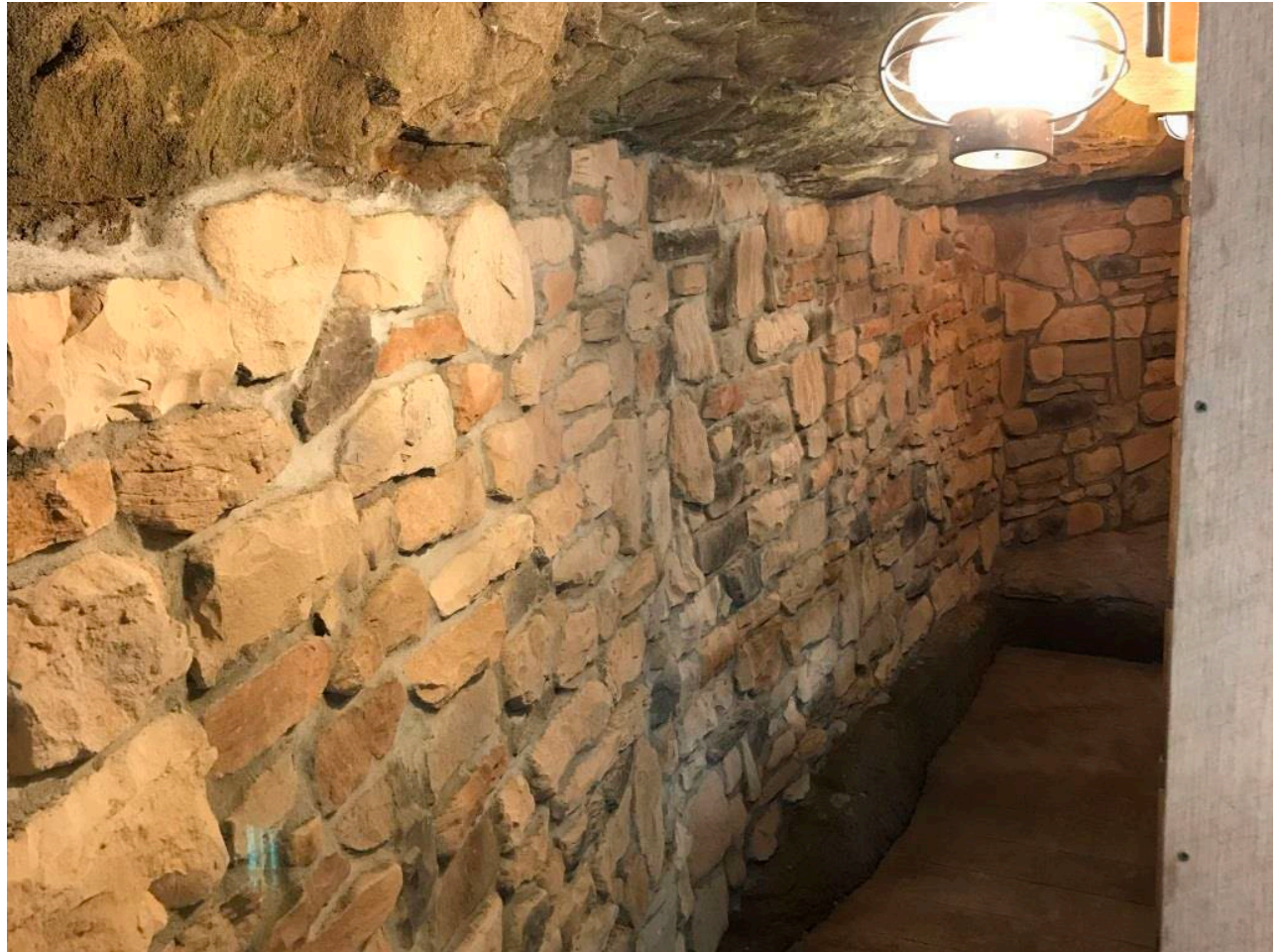
Retaining Wall under Mill | Stebelton Park at Rock Mill
