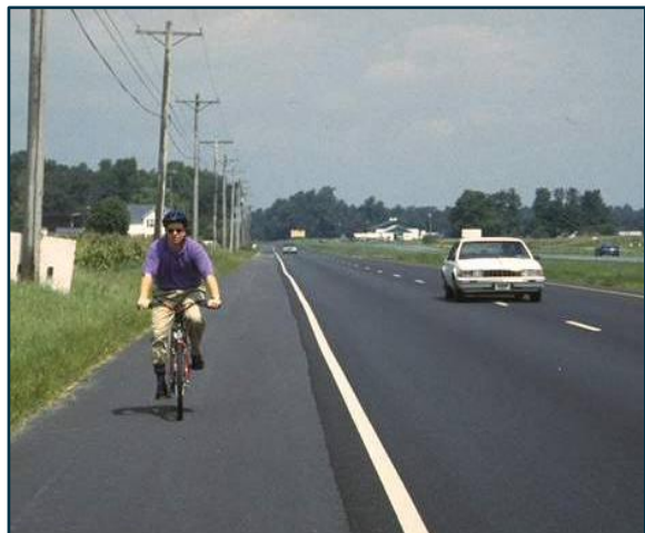
Image 2: Example of a paved shoulder
