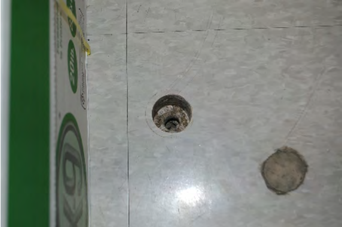
C-5. Hole in floor slab after removal of sub-slab Vapor Pin™ assembly.
