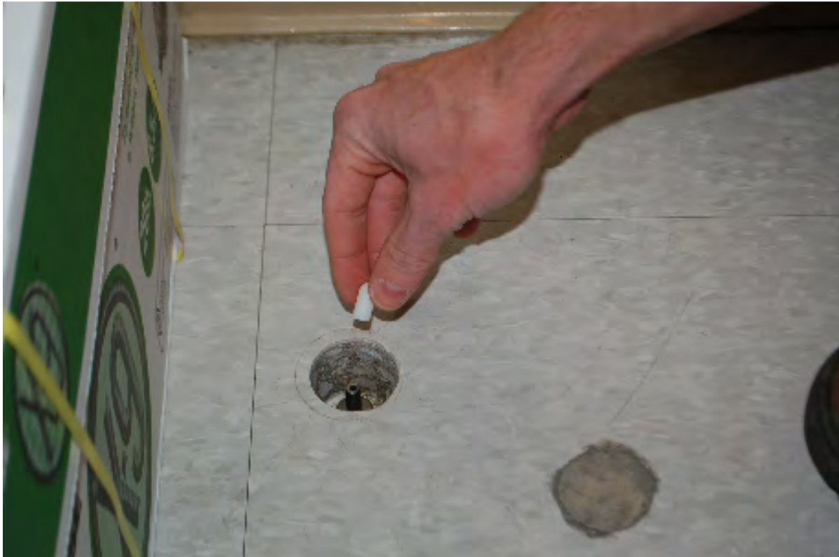
C-2. Removal of the cap from the sub-slab Vapor Pin™ assembly.
