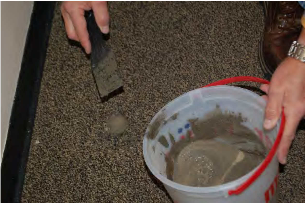
C-6. Filling hole in floor slab with patching cement.
