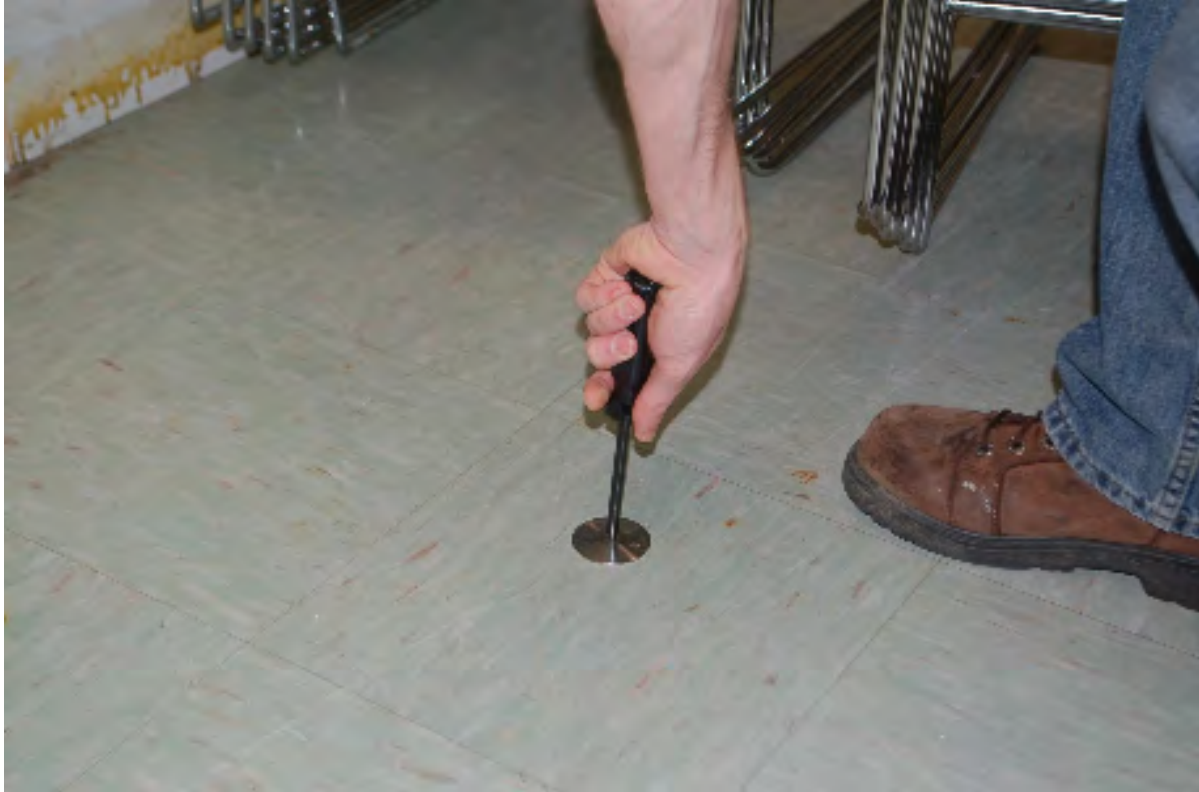
C-1. Removal of the cover plate for the sub-slab Vapor Pin™ assembly with the spanner tool.
