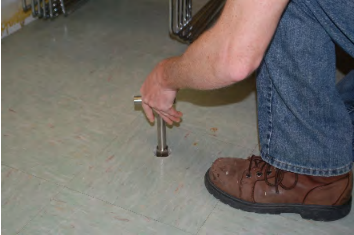
C-3. Using specialized tool to remove sub-slab Vapor Pin™ assembly.
