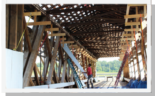
Johnson Bridge under construction
