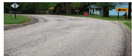
Oberle Ave. to be widened
