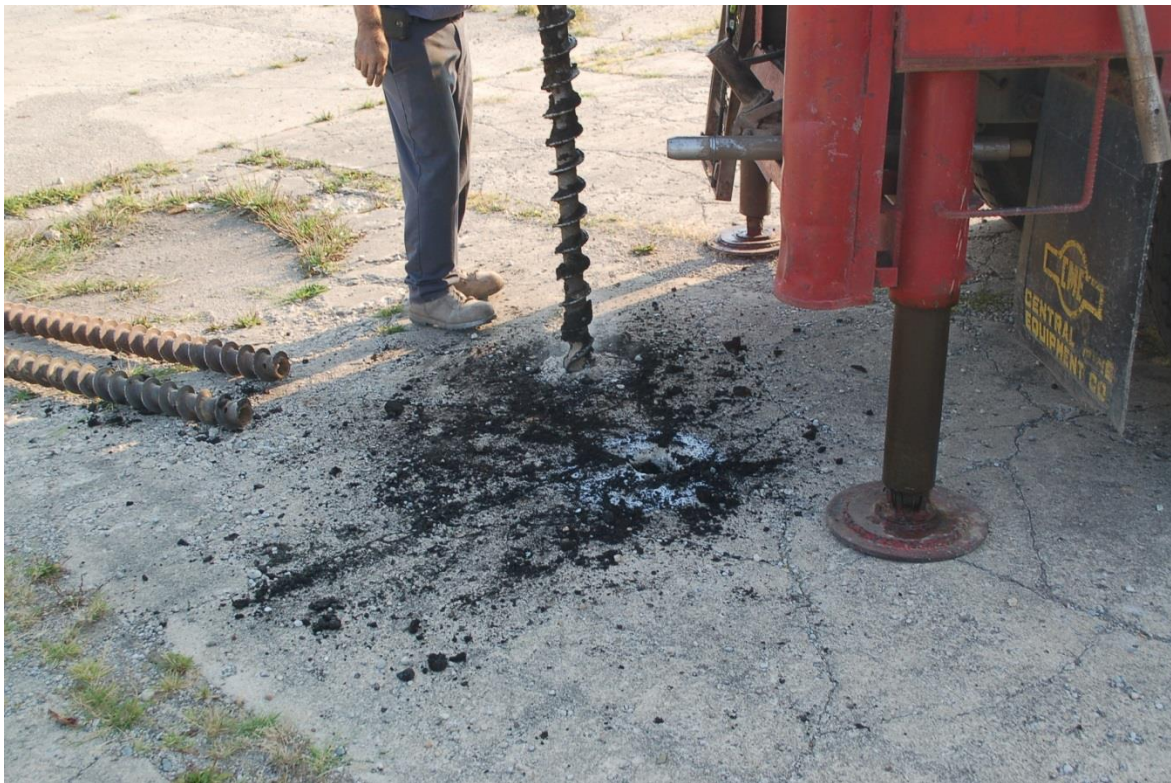
Figure B-2. Solid stem augers on ground waiting to be used in drilling (September 1, 2015).
