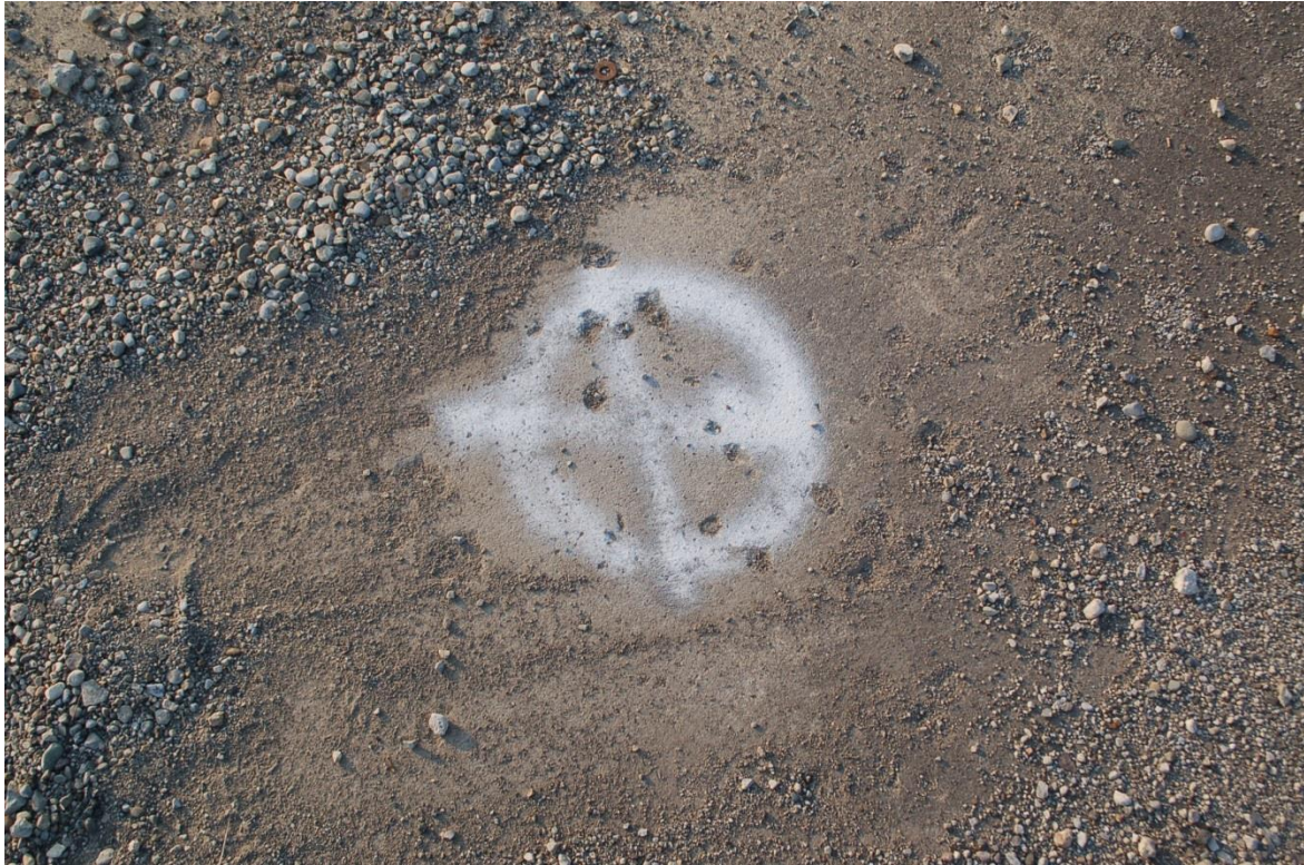
Figure B-1. Markings used to identify boring locations (August 27, 2015).
