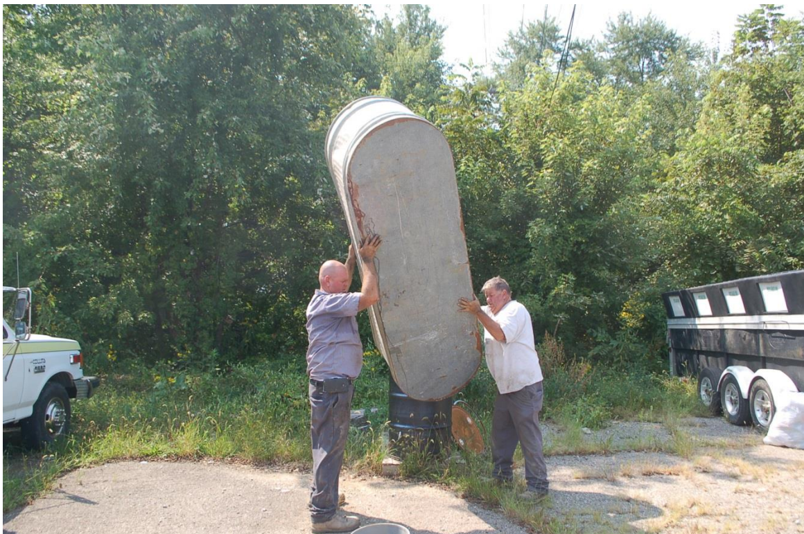
Figure B-6. Emptying the container used to collect decontamination water from the augers into existing onsite barrel containing decontamination water (September 2, 2015).
