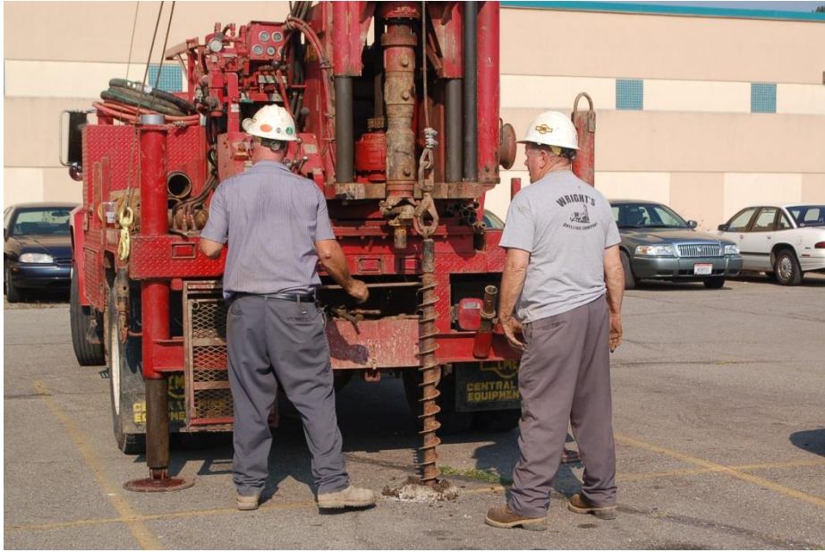
Figure B-3. Drilling using solid stem augers (September 1, 2015).
