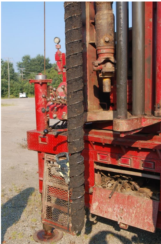
Figure B-4. Cuttings on solid stem augers used to identify depth to bottom of fill materials (September 1, 2015).
