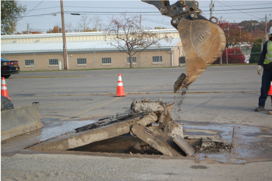
A-3. Removal of concrete and asphalt from excavation (October 27, 2014).
