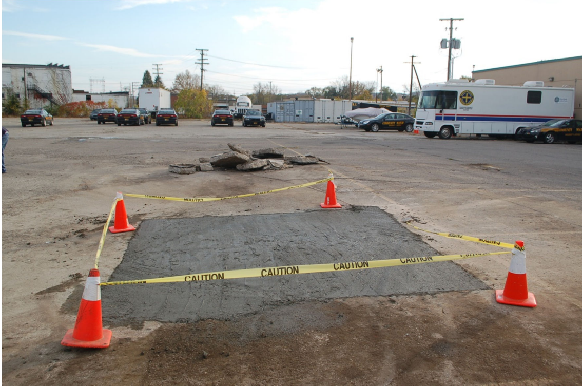
A-13. Excavation filled with concrete and surrounded by cones and caution tape (October 27, 2014).
