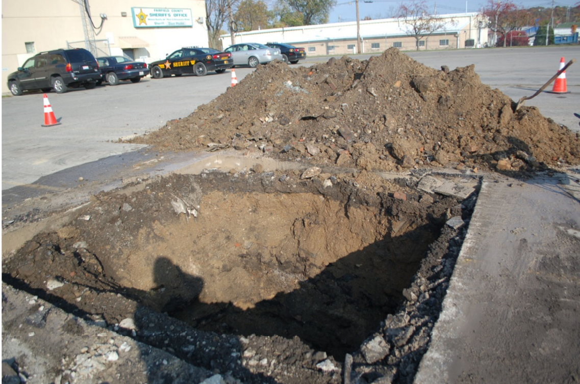
A-5. Excavation and stockpiled fill materials (October 27, 2014).
