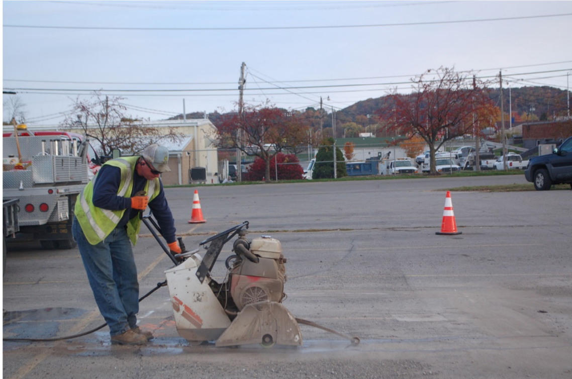
A-2. Cutting concrete with gas-powered saw (October 27, 2014).
