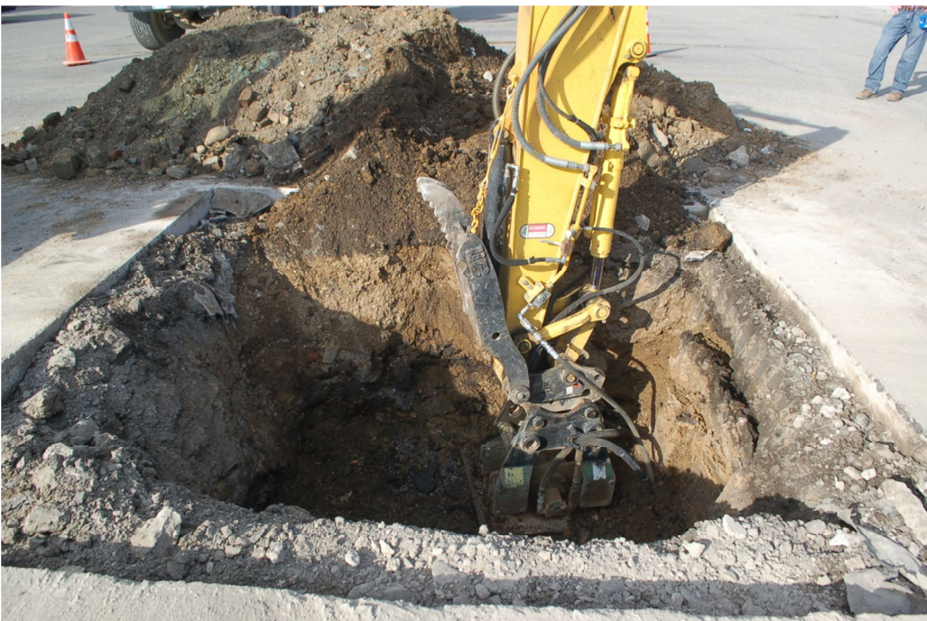
A-8. Compaction of fill materials during filling (October 27, 2014).
