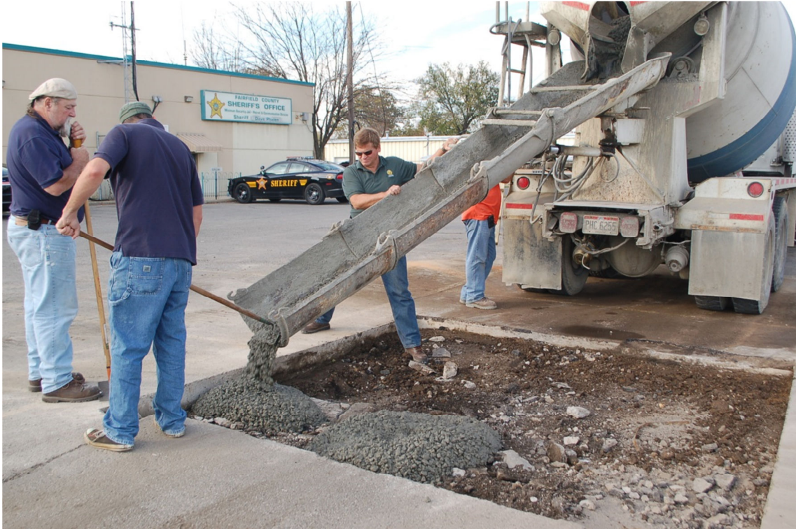
A-12. Filling top six inches of excavation with concrete (October 27, 2014).
