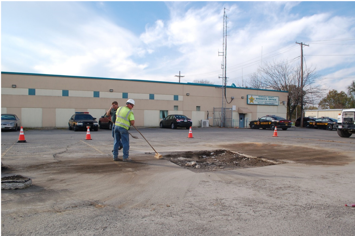
A-10. Excavation re-filled and surrounding concrete broom cleaned (October 27, 2014).
