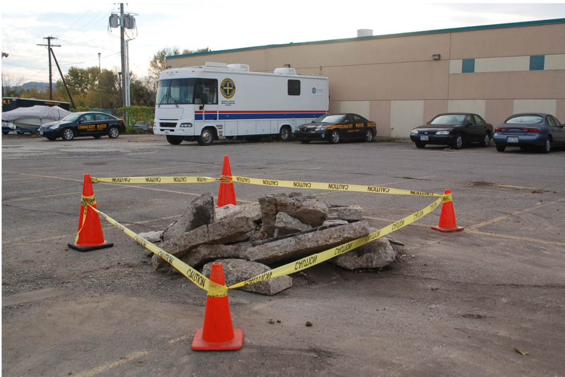
A-14. Remaining surface concrete with cones and caution tape prior to moving to western portion of the site (October 27, 2014).
