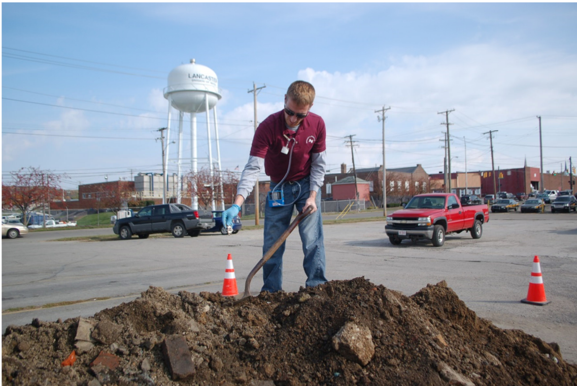
A-6. Fill material manipulation after excavation complete (October 27, 2014).
