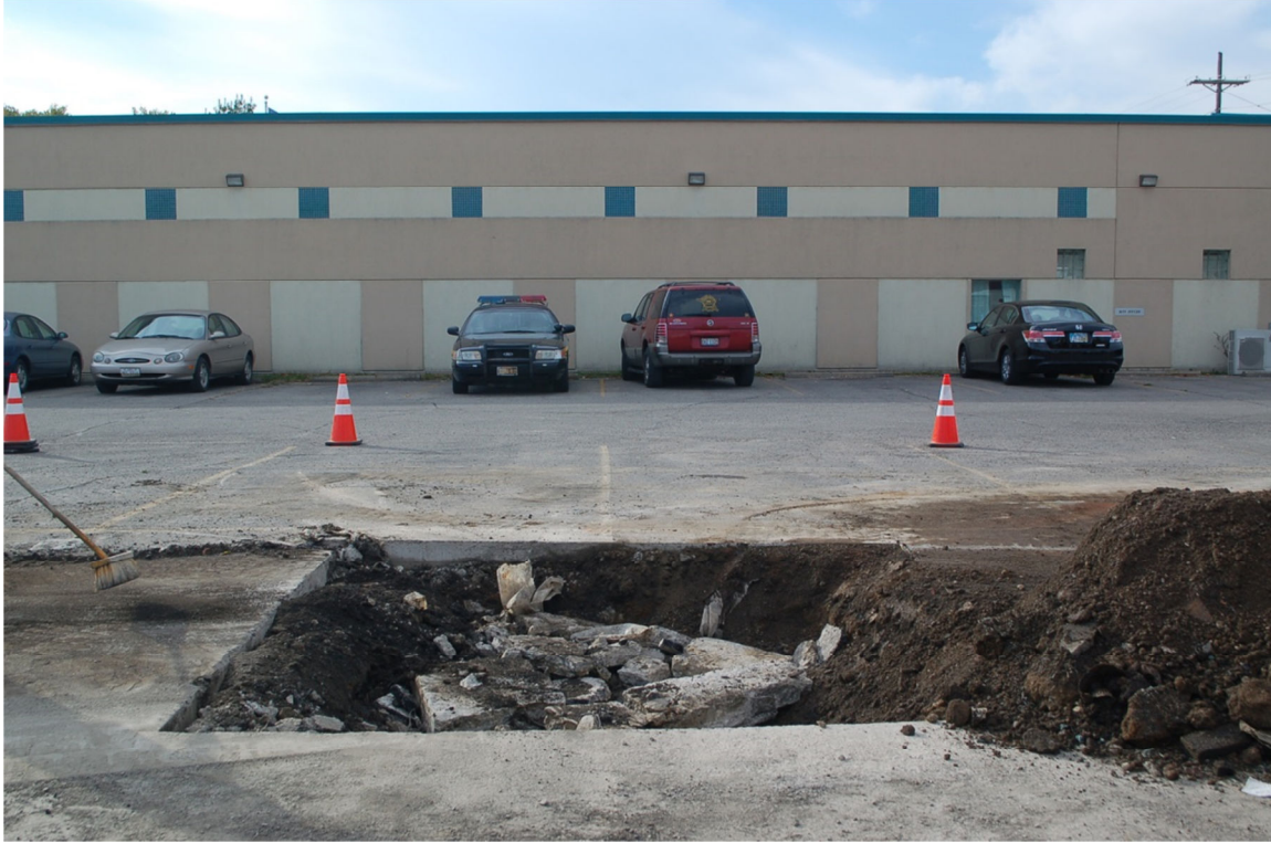
A-9. Surface concrete and asphalt placed in excavation (October 27, 2014).
