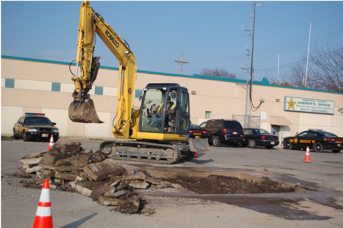
A-4. Surface concrete and asphalt stockpiled during excavation (October 27, 2014).
