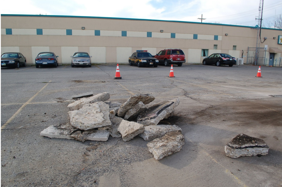
A-11. Remaining concrete and asphalt that could not be placed in the excavation (October 27, 2014).
