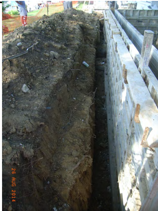
BUCKEYE LAKE 25 AUGUST 2014 Photo 044 – Unsupported excavation into embankment.
