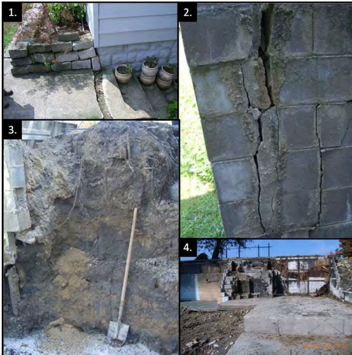
Figure 1. Typical Embankment Distress Observations 1) Differential settlement of structure built into crest/embankment longitudinal cracking 2) Failing masonry unit wall supporting landside embankment materials 3) Unsupported excavation into downstream face of embankment which could cause weakening of embankment soils and embankment failure 4) Several rows of masonry unit walls were noted in old house foundations likely indicating seepage related displacement
