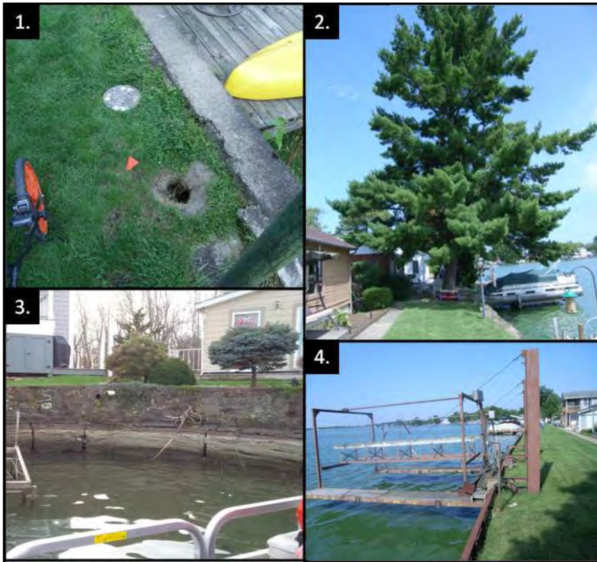
Figure 2. Typical Distress Observations 1) One of many depressions behind masonry wall 2) Tree with root system spanning the entire embankment crest 3) Numerous cracks within base of, and pipe/utility penetrations through, masonry wall observed during winter pool drawdown 4) Dock structures cantilevering from the dam put stress on the sheetpiling for which it was not designed
