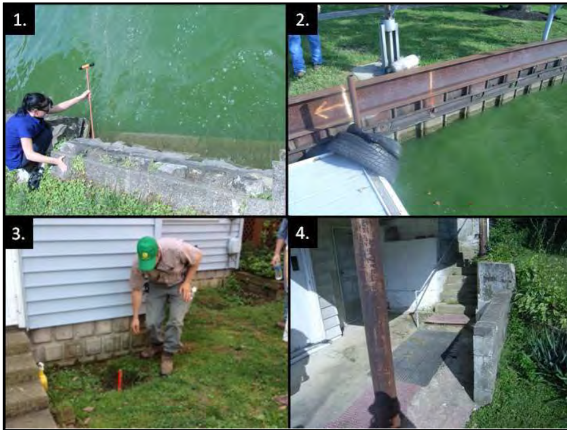
Figure 3. Other Wall and Seepage Observations 1) Displaced portion of masonry wall 2) Numerous rust holes observed in sheetpiling 3) Several depressions possibly due to boils, together with very shallow ground water conditions, were observed 4) Location of persistent seepage near Black Diamond Point
