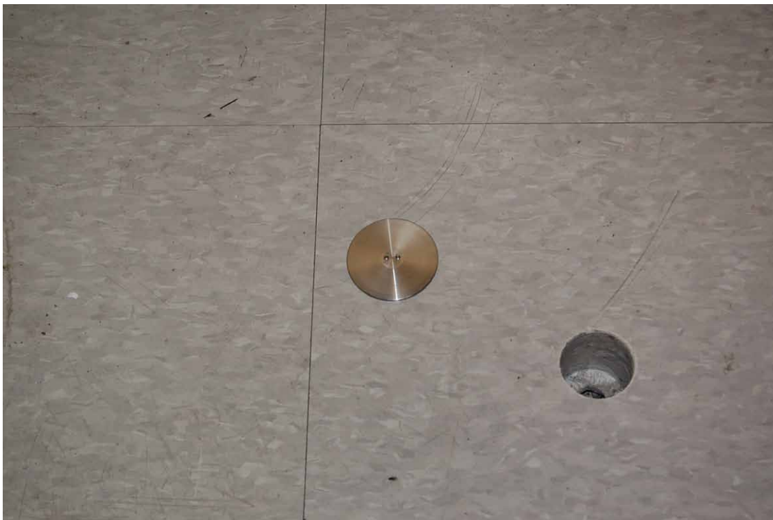
C-6. Completed Vapor Pin™ installation (left) with flush-mounted protective cover and drilled hole where subsurface wrapped wire cable prevented installation of Vapor Pin™ prior to filling (July 18, 2014).
