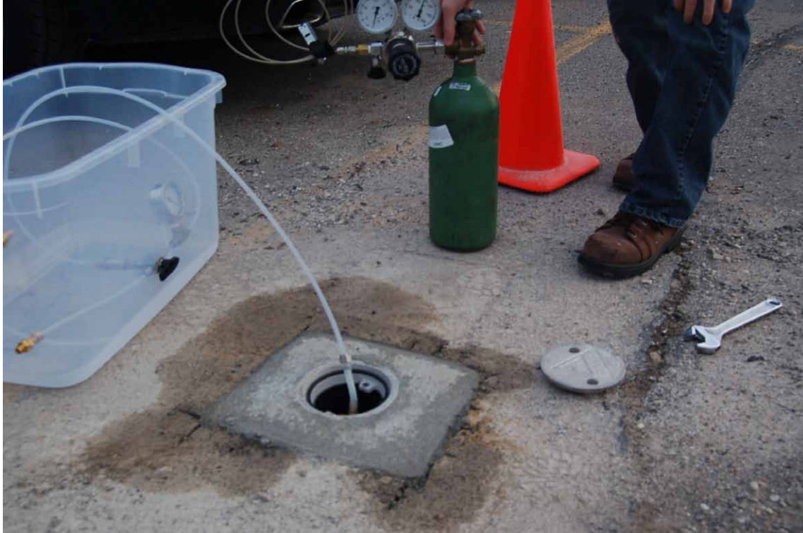
D-1. Connecting tubing to subsurface soil gas probe in preparation for integrity testing with shroud at left (July 24, 2014).
