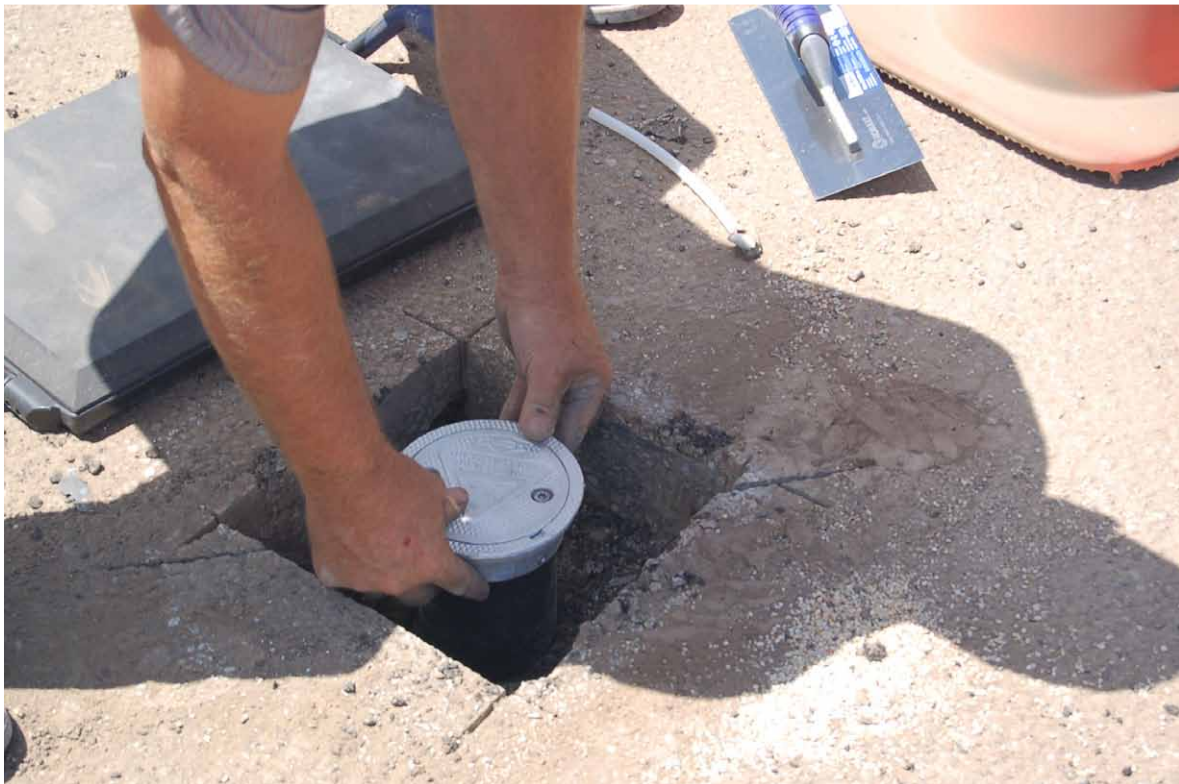
B-8. Installing surface protector around petcock (July 17, 2014).
