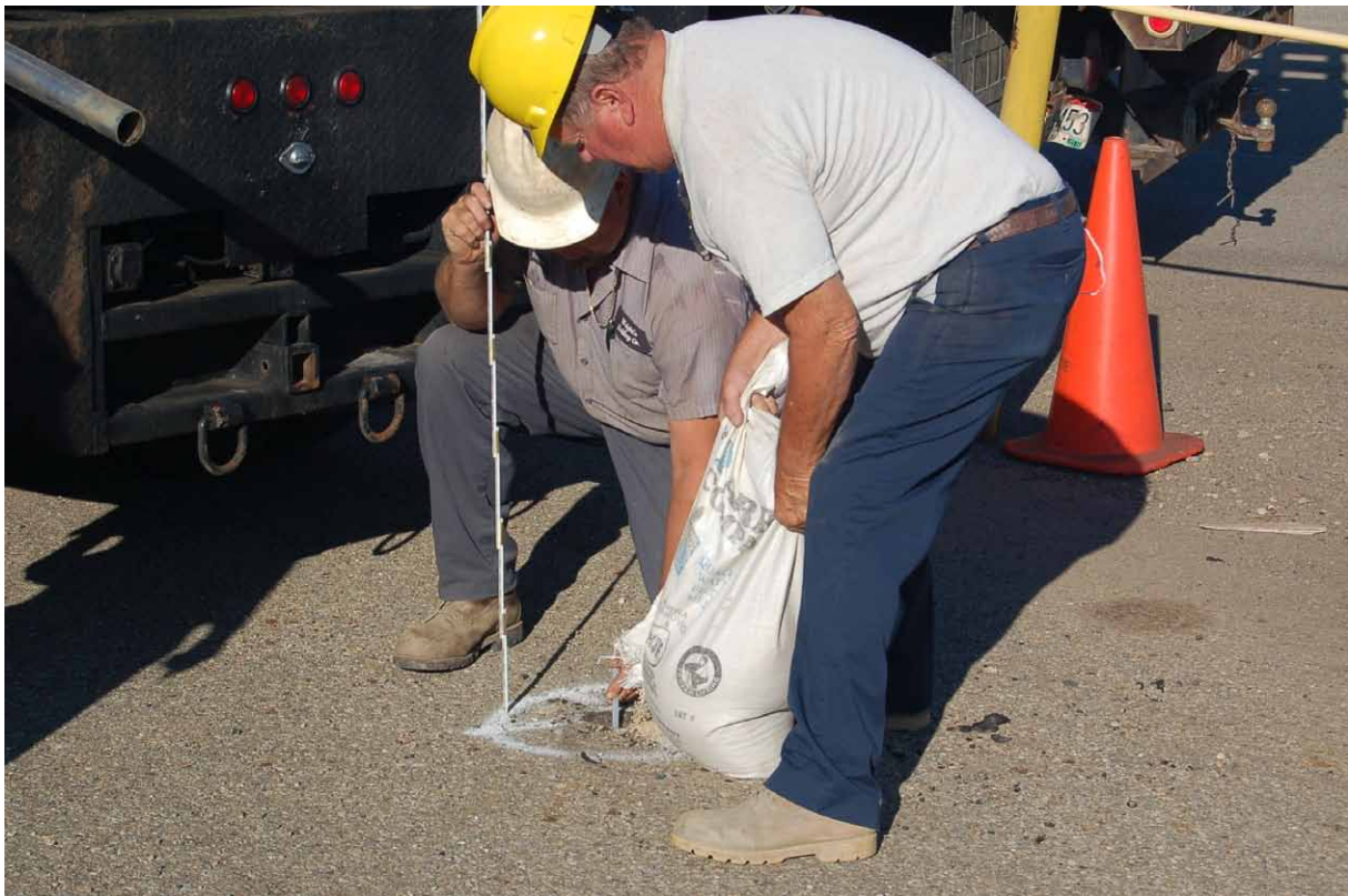
B-4. Installing sand pack around Teflon® tubing and vapor point (July 17, 2014).
