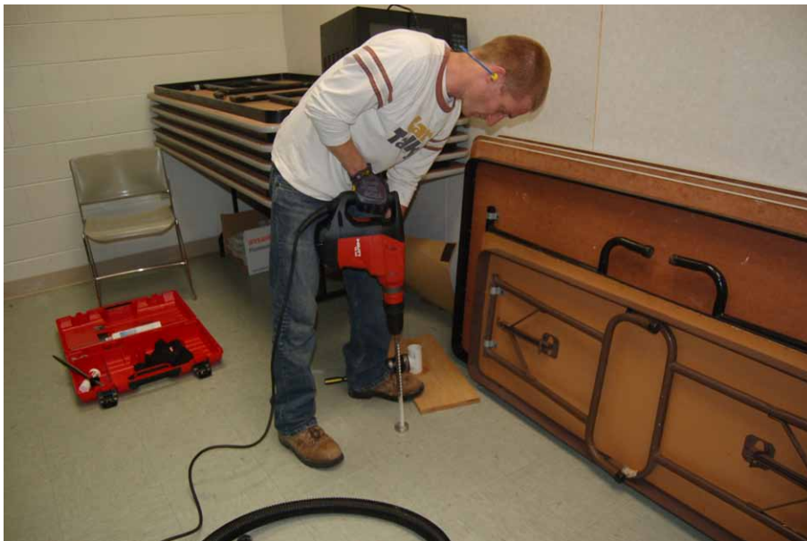
C-2. Drilling 5/8-inch hole through concrete slab using drilling guide (July 18, 2014).
