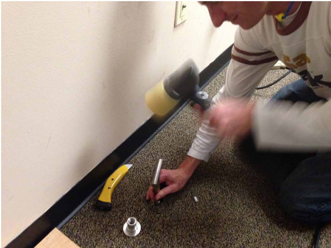
C-4. Installing Vapor Pin™ in drilled hole in concrete slab (July 18, 2014).
