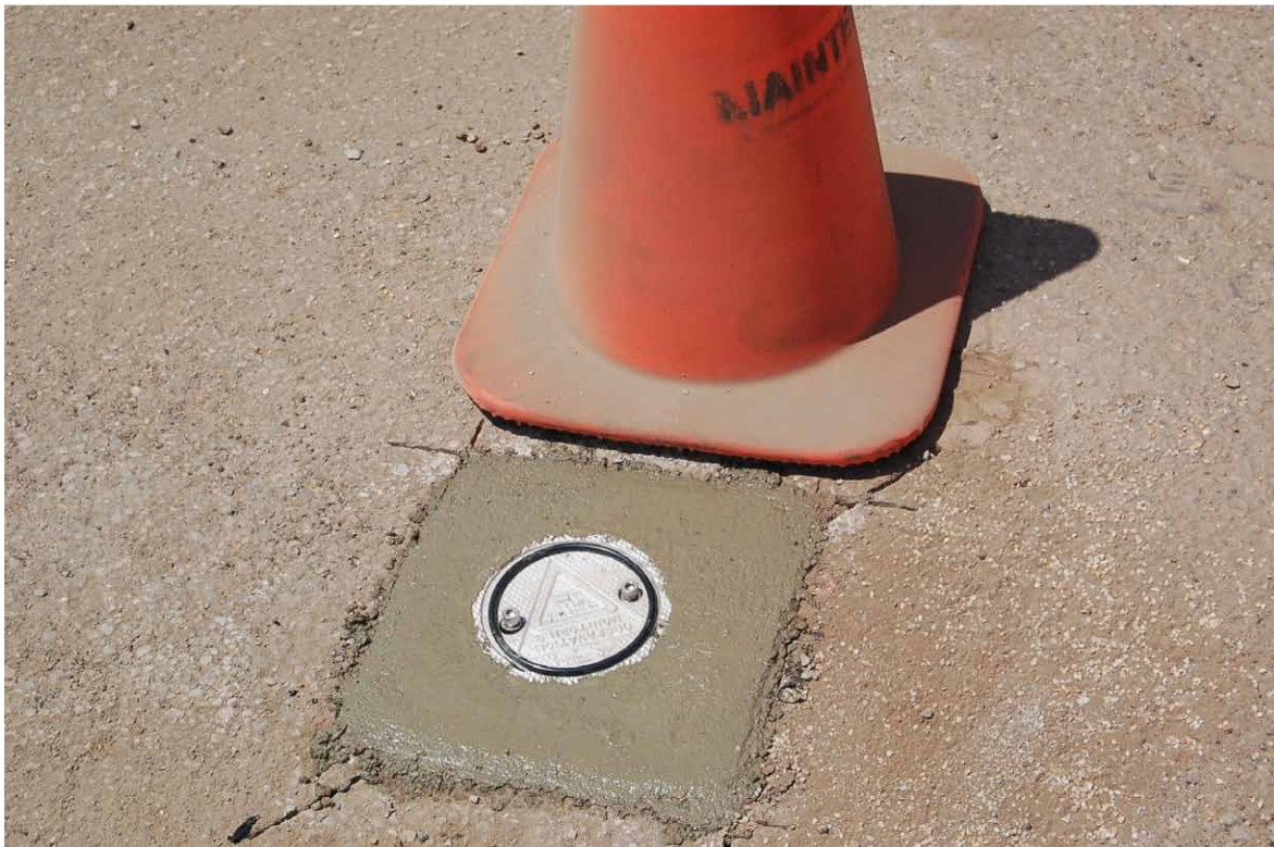
B-10. Completed subsurface soil gas sampling point (July 17, 2014).
