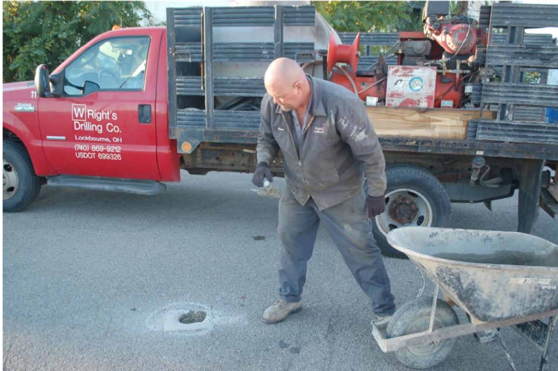
H-5. Adding Quickrete to former subsurface gas probe location (September 24, 2014).
