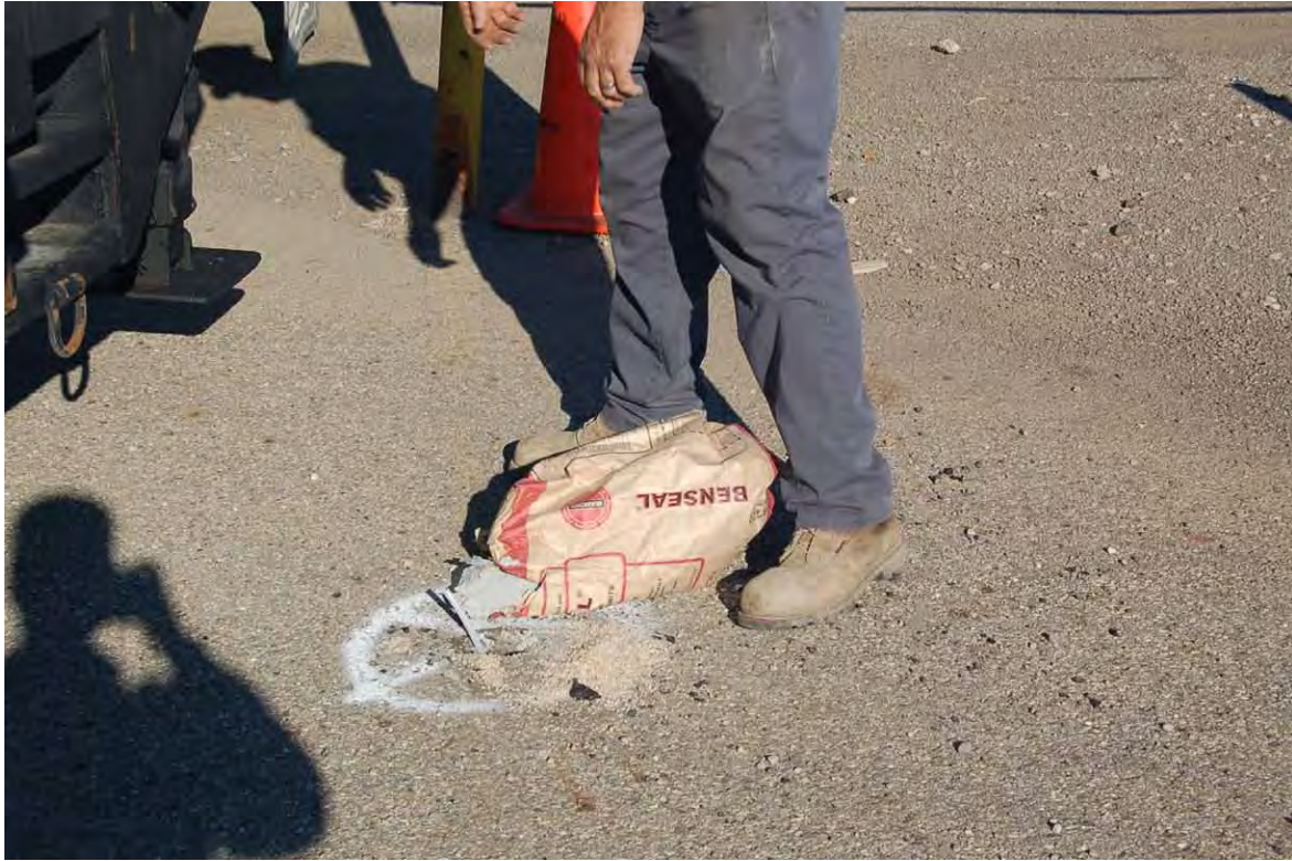
B-5. Ready to install Benseal above the sand pack (July 17, 2014).
