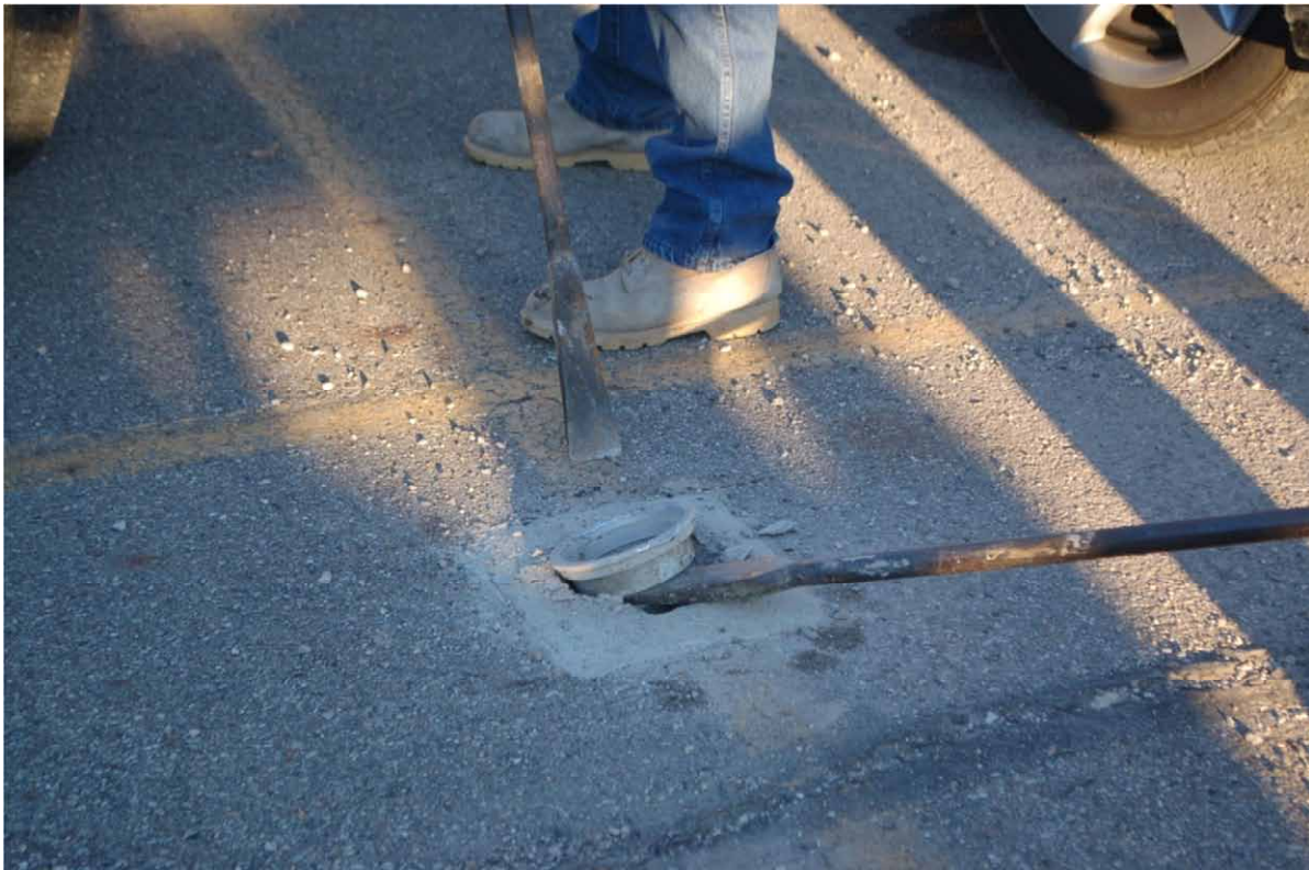
H-4. Removing metal ring portion of the protector (September 24, 2014).
