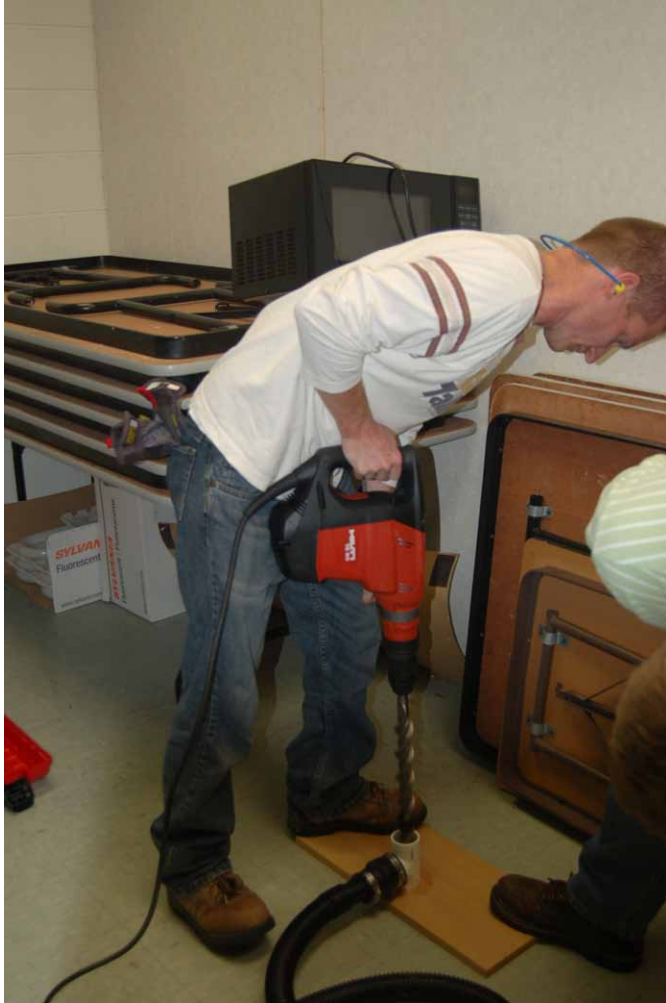
C-1. Drilling a shallow 1 ½ -inch diameter outer hole in the concrete slab (July 18, 2014).
