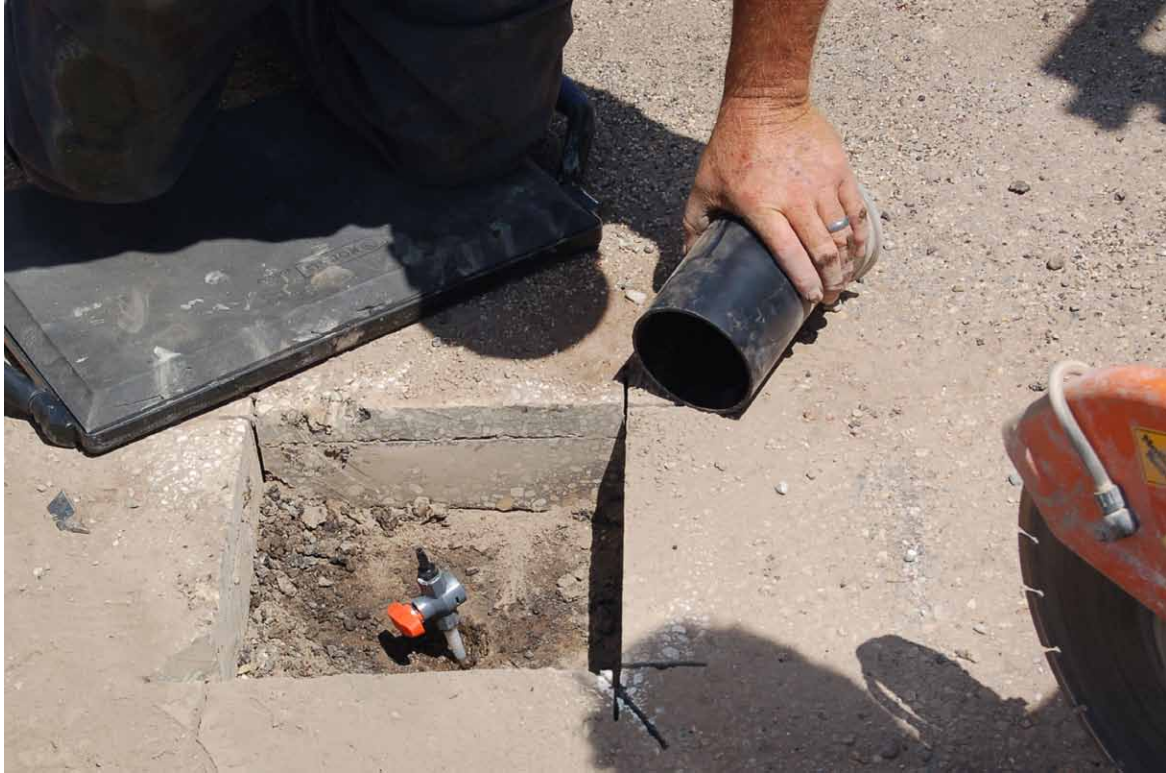
B-7. Petcock attached to top of Teflon® tubing and surface protector ready for installation (July 17, 2014).
