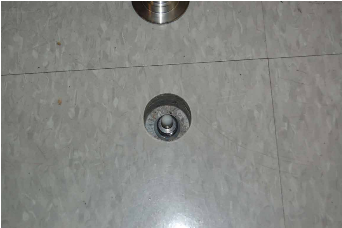
C-5. Installed Vapor Pin™ with cap on top (July 18, 2014).
