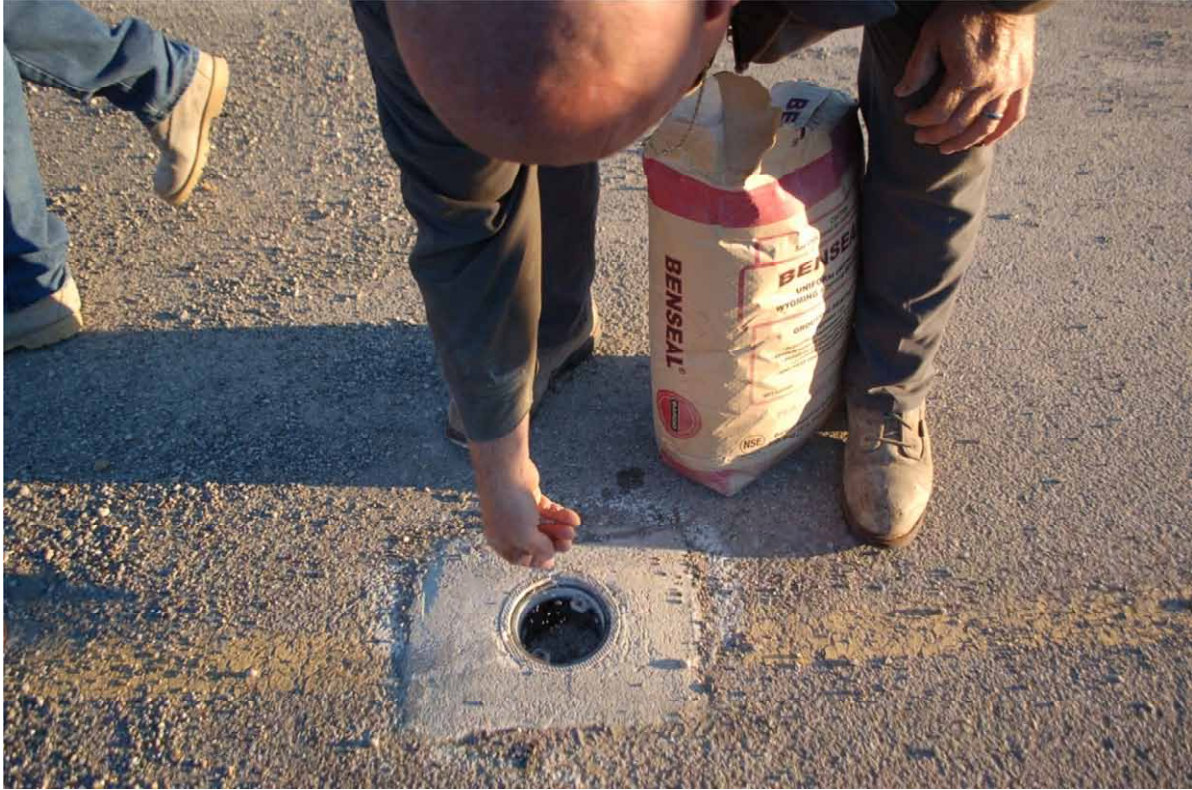
H-3. Adding Benseal to fill place where tubing was removed (September 24, 2014).
