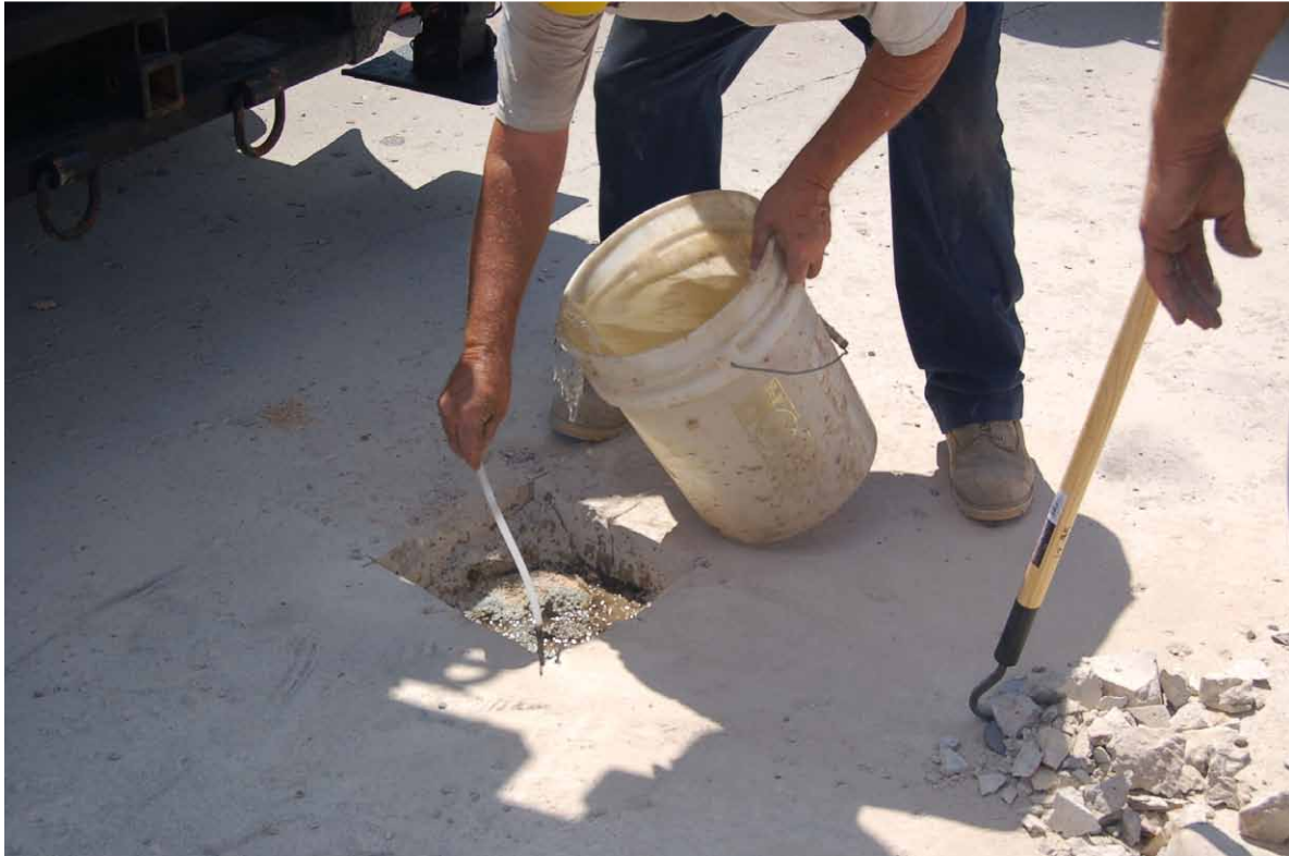
B-6. Hydrating Benseal after placement (July 17, 2014).
