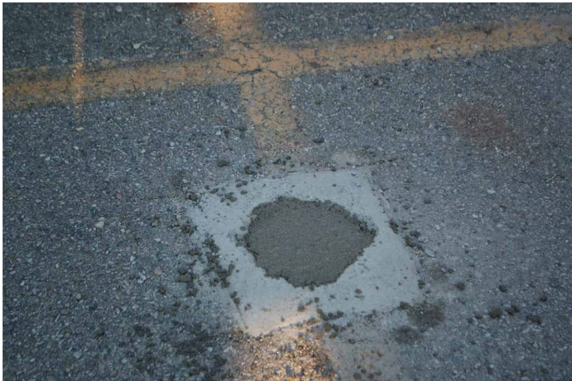
H-6. Completed abandonment of subsurface gas probe (September 24, 2014).
