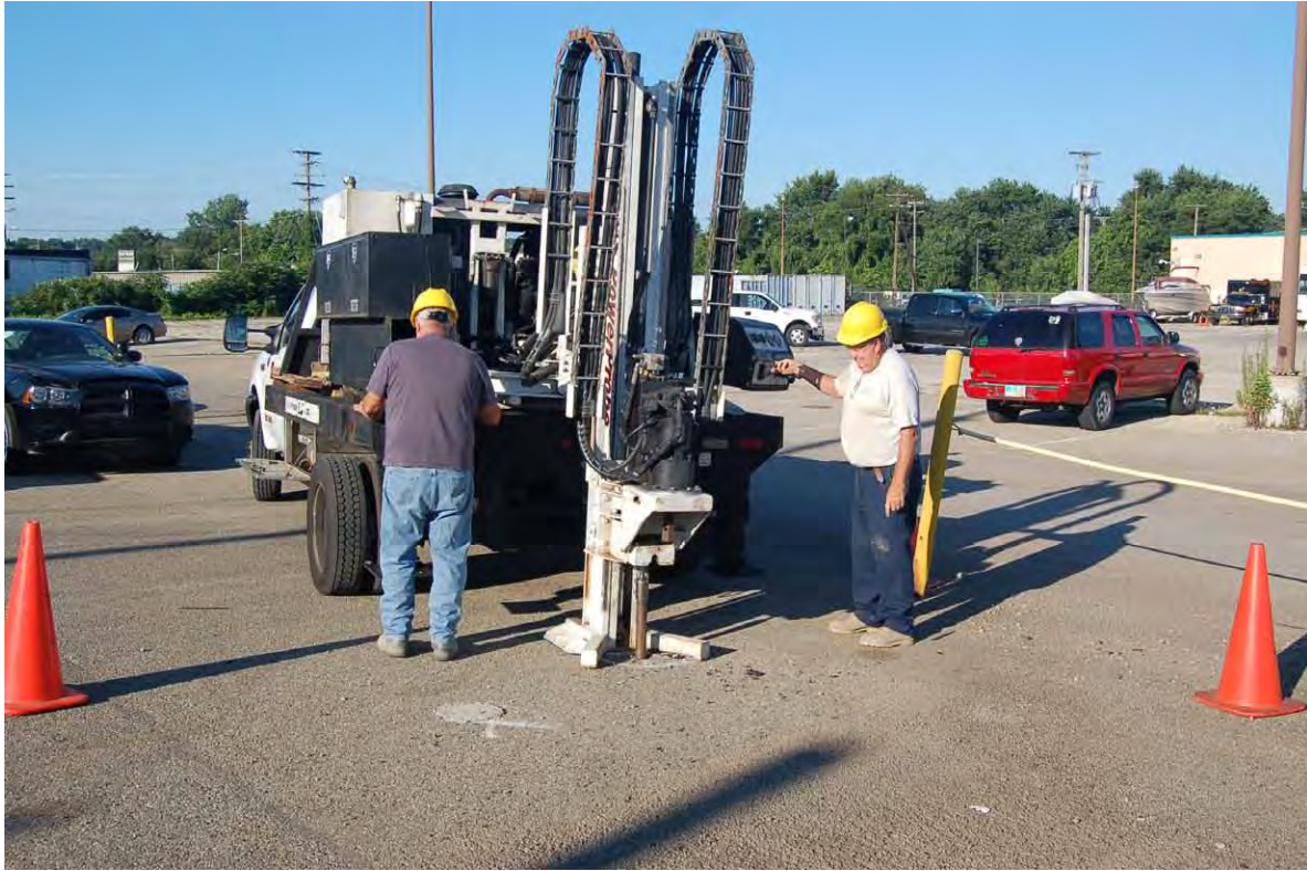
B-1. Drilling rig advancing rods to desired depth (July 17, 2014).
