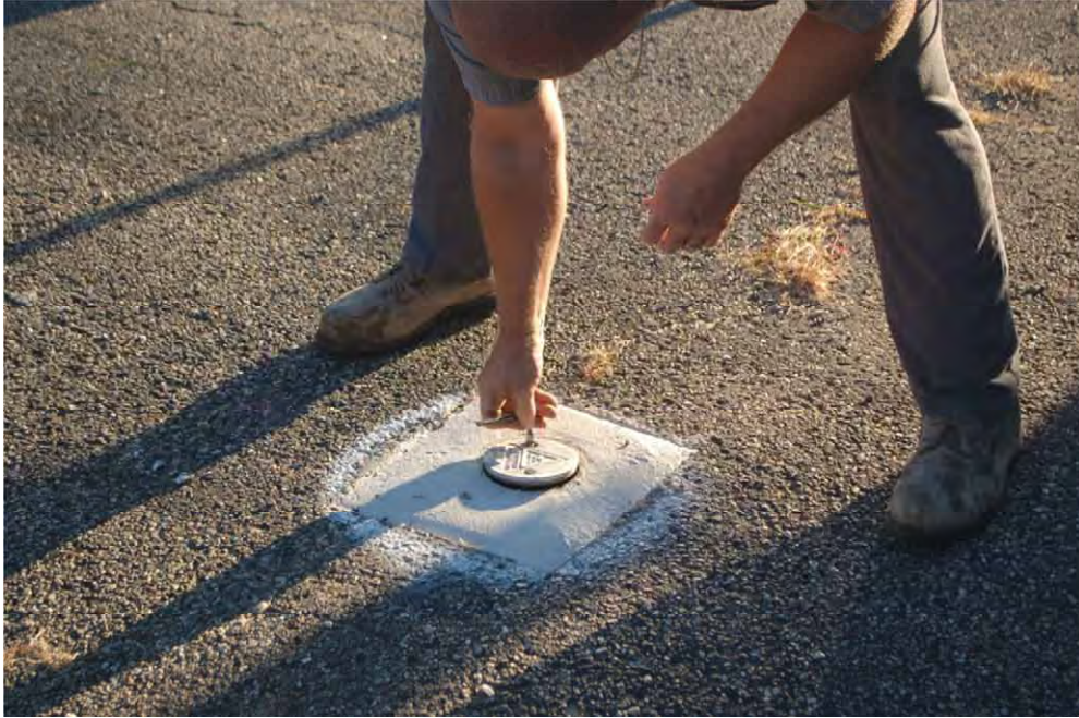
H-1. Removal of protective cap prior to abandonment of the subsurface gas probe (September 24, 2014).
